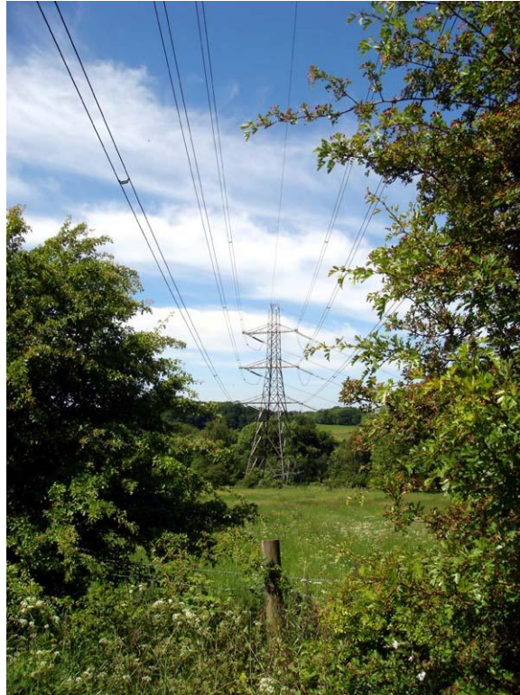
Photo 1 - Sample Caption - Power lines near sample customer
