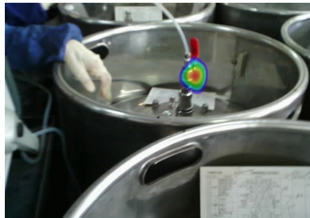
Gas pipeline leakage
